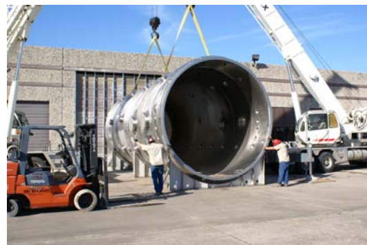
Chamber installation, new Houston Facility
