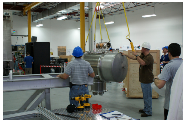
VX-200 Superconducting magnet arrival and installation at Ad Astra’s Houston facility
